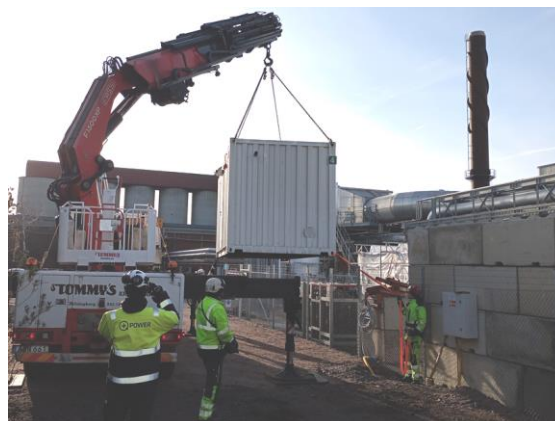
Figure 2. The biological methanation plant is lifted in place. Photo: Jörgen Held.
